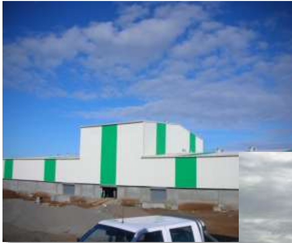
Civil Structures Building
